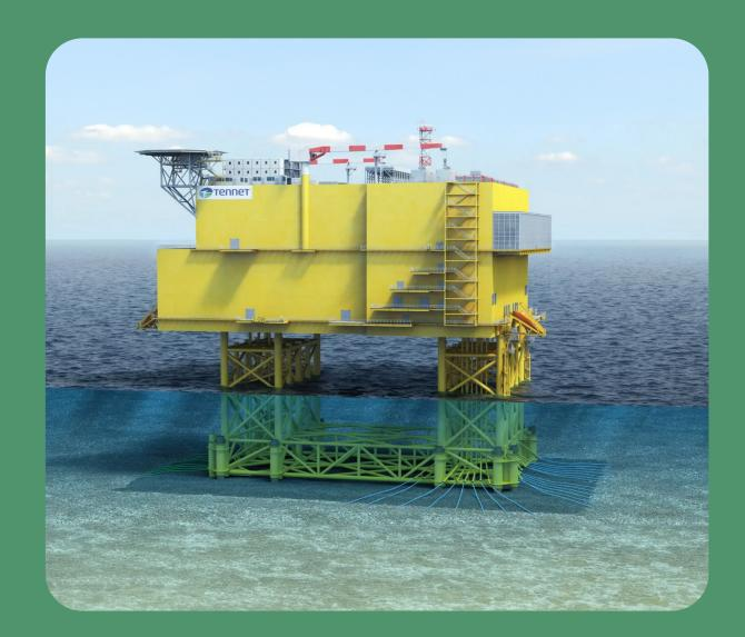
We embarked on two major projects that support TenneT's ability to provide electricity to European markets from windfarms in the German North Sea. In 2023, we initiated fabrication, transportation, and installation support for the topside module of TenneT's BorWin6 980MW high-voltage, direct current (HVDC) project.
