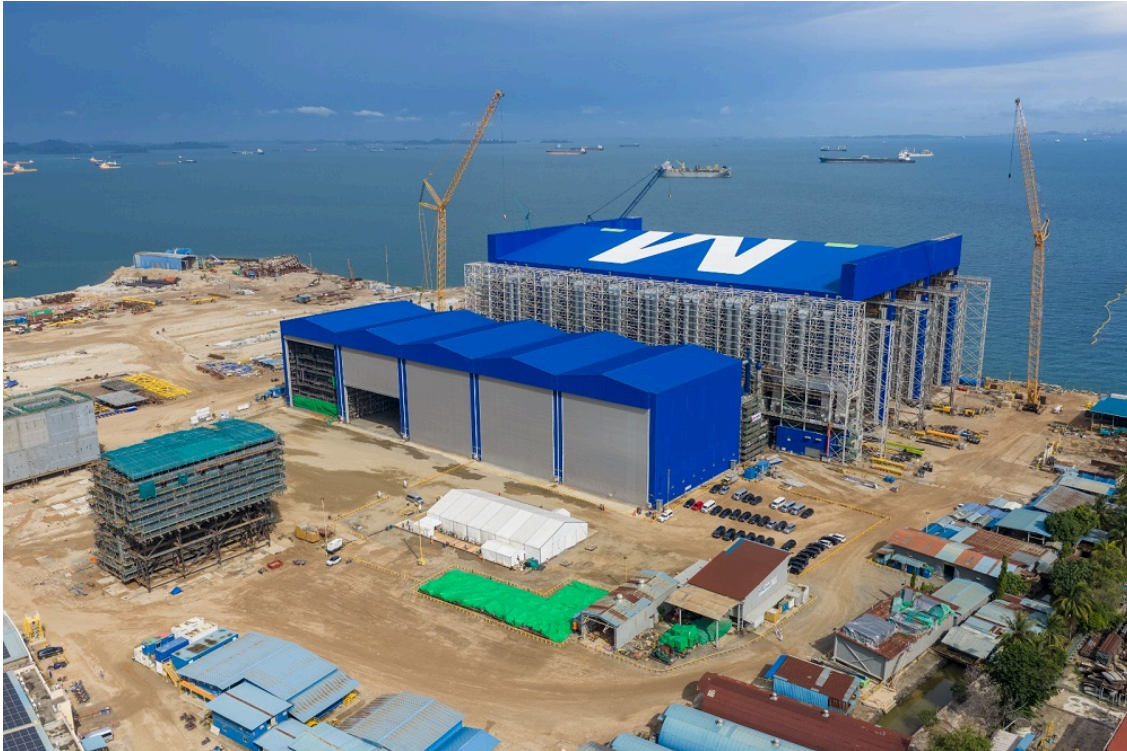
McDermott inaugurates the Cakrawala and Nusantara Buildings at its Batam Fabrication Yard to support global offshore wind energy projects. Photo: McDermott's Batam
