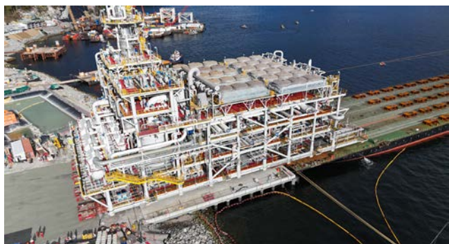
Figure 2. Recent mega-module load-out from McDermott's module yard using a self-propelled modular transporter system.
