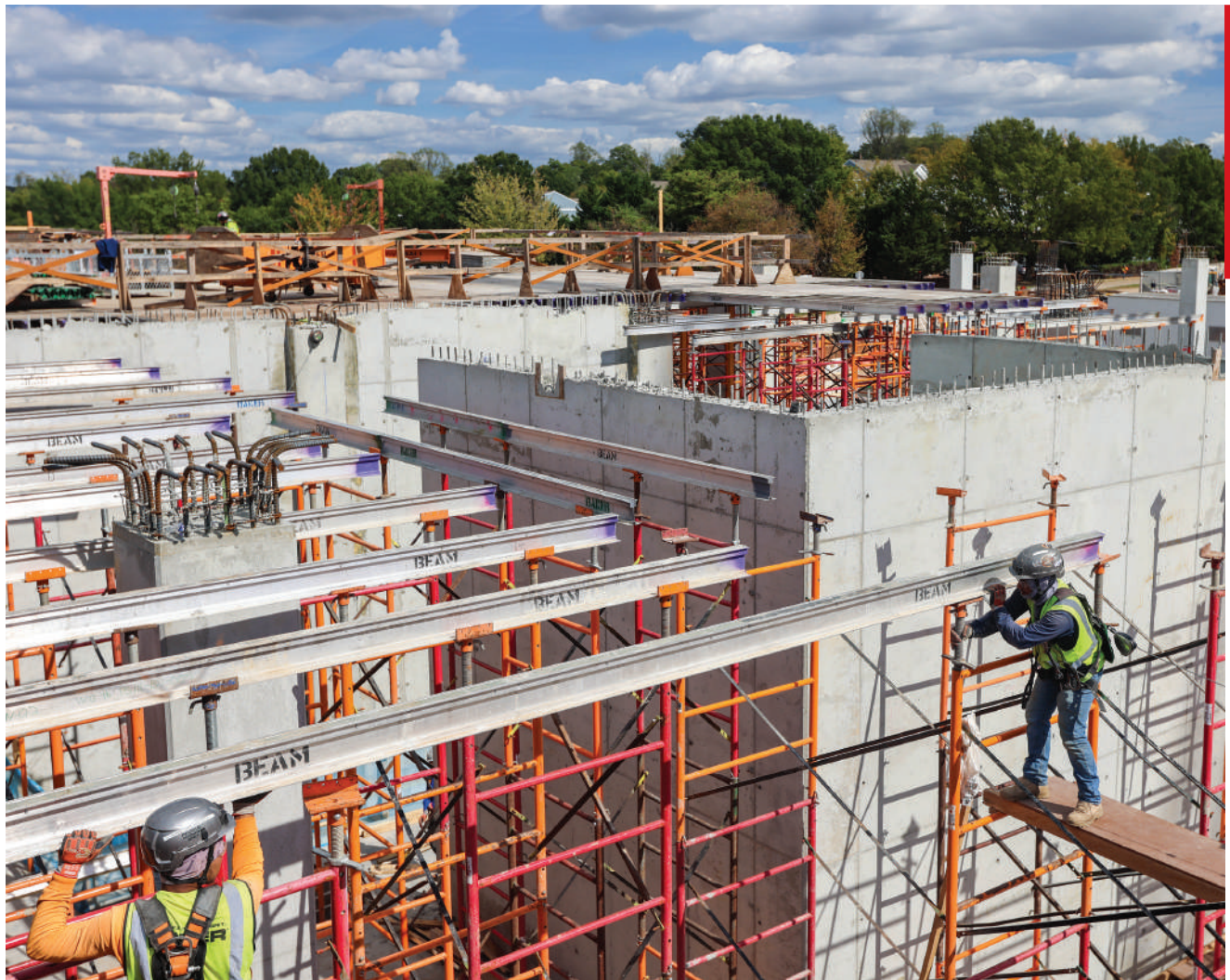
PHOTO COURTESY OF HITT CONTRACTING
