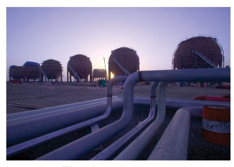
CB&I pioneered the concept of field-welding spheres in the 1920s and built the world's first field-erected Hortonsphere vessel in 1923. Since then, we have designed and built thousands of spheres around the world, including liquid spheres up to 94 feet (28.6 m) in diameter and gas spheres up to 110 feet (33.5 m) in diameter. We built the world's largest self-supporting sphere, measuring 225 feet (69 m) in diameter nuclear plant containment vessel in New York.
