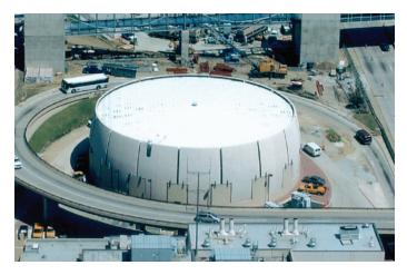
SoCool fluid can match or exceed the resulting power output increase of other TIC systems, while retaining the simplicity, reliability, efficiency and rapid discharge benefits of stratified water TES at installed costs as low as \$300, or less, per kW of net power enhancement.
