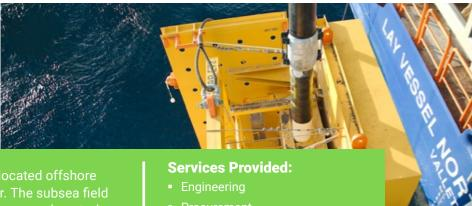
The Siakap North-Petai (SNP) field is located offshore Sabah, Malaysia, in 4,429 feet of water. The subsea field development consists of subsea hardware and controls, two rigid, insulated, pipe-in-pipe production flowlines, one rigid water injection flowline and one main umbilical system connecting eight new manifolds and subsea distribution units to existing riser slots in the Kikeh FPSO
