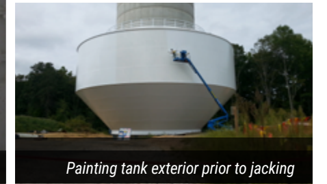
Jacking a 2,000,000 gallon tank in Whitestown, IN
