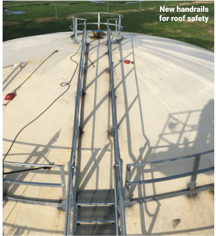
In-tank valve installation
