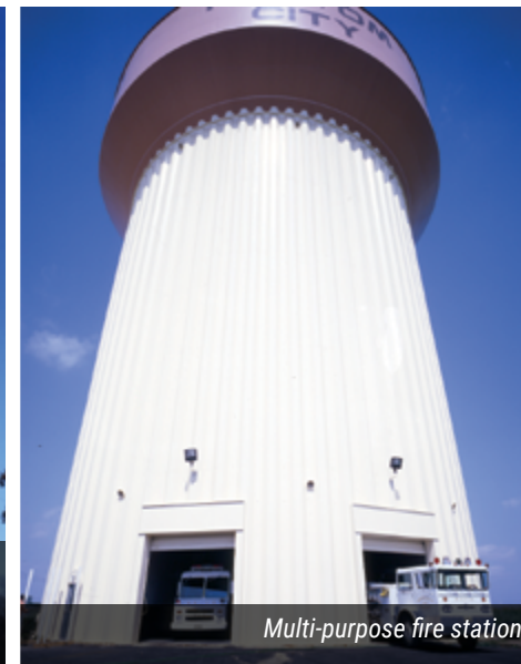
Dual storage - 620,000 gallons upper tank and 1,130,000 gallons lower tank; (STI/SPFA Tank of the Year)
